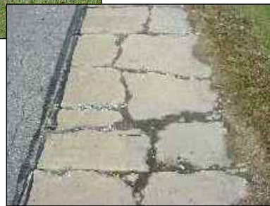
ANY SIDEWALK BLOCK (BASED ON 20 SQ. FT.) HAVING A CRACK OR CRACKS IN IT OF AT LEAST 1/2 INCH WIDE WITH A MINIMUM OF 4 LINEAL FEET IN ONE BLOCK. (VARIOUS SIZE BLOCKS WILL BE EVALUATED PROPORTIONALLY.)
