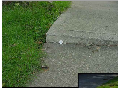
ADJOINING BLOCKS OR PORTIONS THEREOF WHOSE EDGES DIFFER VERTICALLY BY MORE THAN 3/4 INCH.
