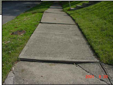
ADJOINING BLOCKS OR PORTIONS THEREOF WHOSE EDGES DIFFER VERTICALLY BY MORE THAN 3/4 INCH.
