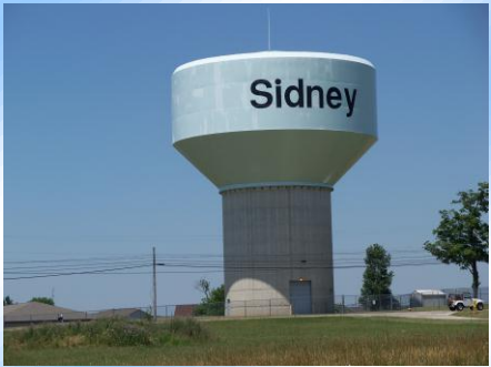
Fourth Street Tank (2MGD)
