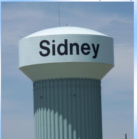
Campbell Road Tank (1 MGD)
